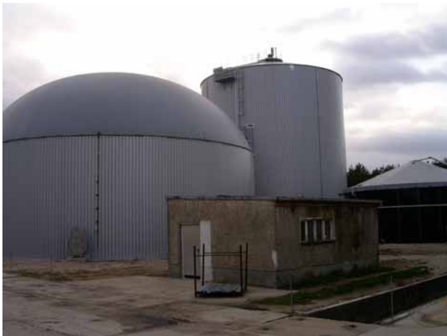
Fig. 5 Digester (background center) and gas storage tank (left) of the biogas plant Sandbeiendorf
